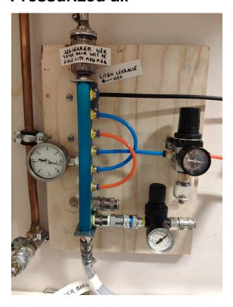
The pneumatic hoses that are used are 6mm diameter
